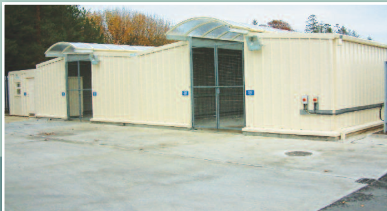
Acute hospital waste storage facility
